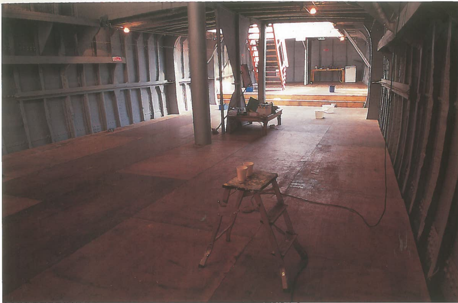
↑ The hold on the SS Robin, which will become the gallery space. All photographs © Alexandra Murphy.
